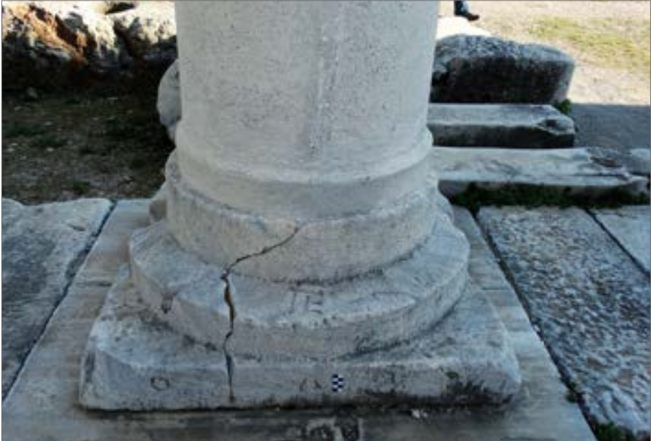
Fig. 7. Ephesos, basilica of St. John, column base with assembly/positioning and workshop marks (Photo G. Marsili)
