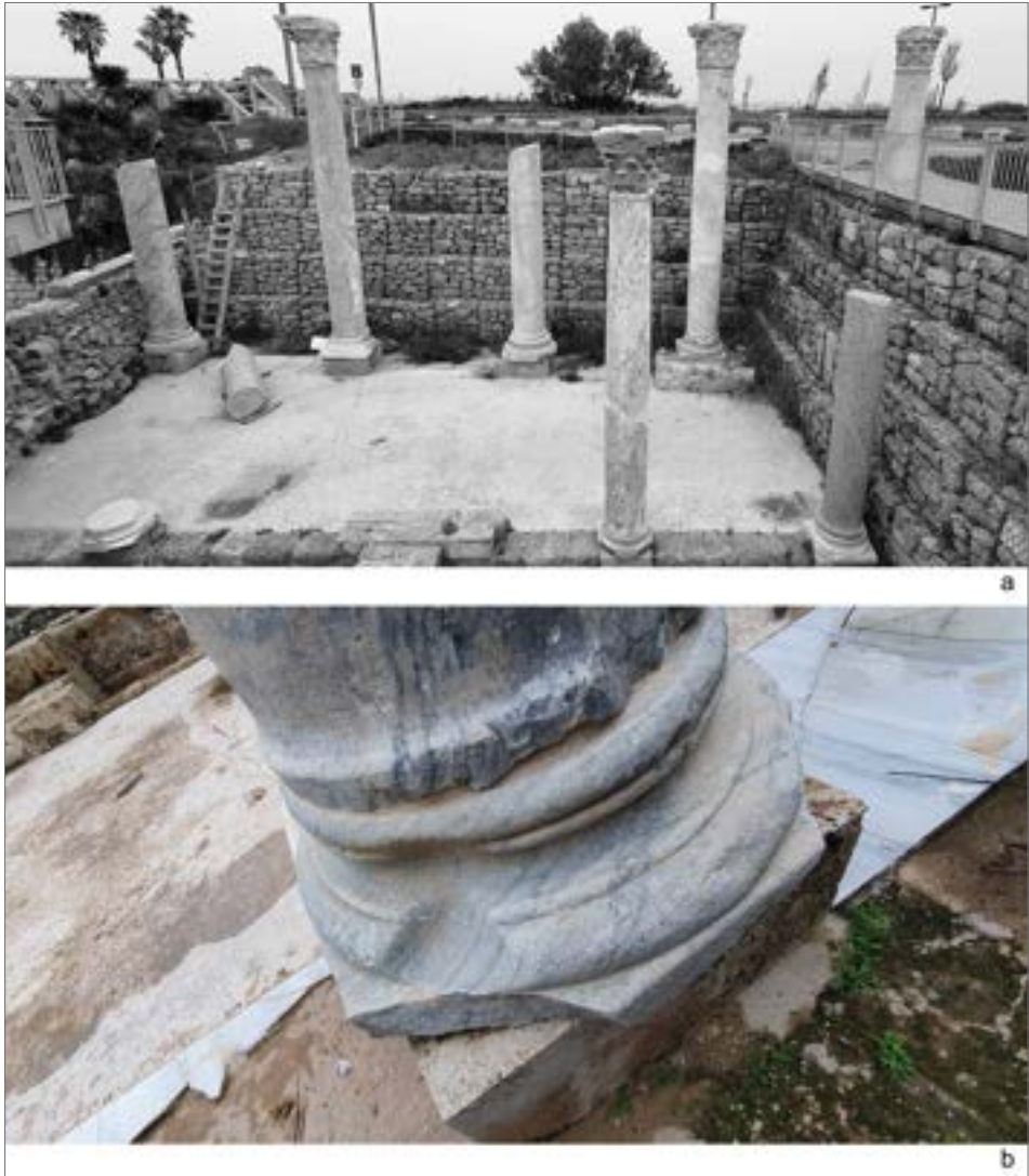
Fig. 13. Late 5th century AD portico: a – general view (IAA | photo A. Peretz); b – Attic-type base with a depression (Photo P. Gendelman)
