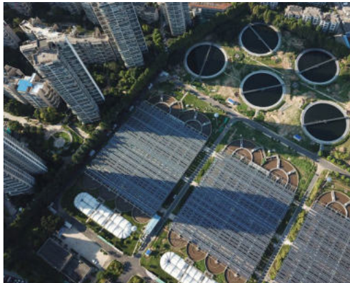
Figure 5: Photovoltaic application in waste water purification.
