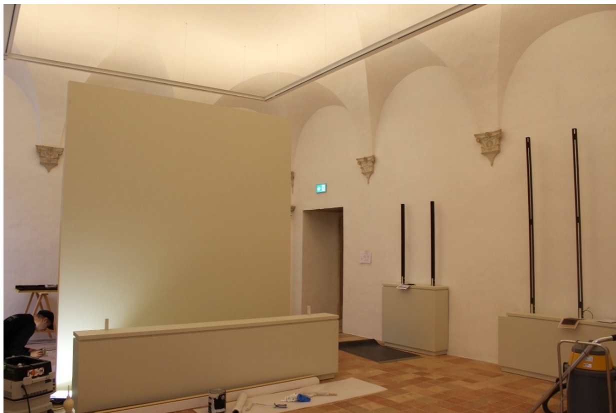
132 Room 148 during renovation, 2024 (A. Fapanni)
