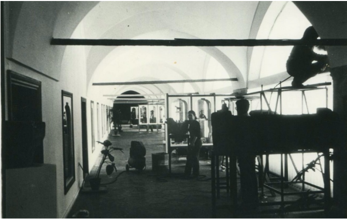
Figure 119. A view of the corridor of TİEM during the opening preparations in 1983. Source: Hüsrev Taylan Archive in Atatürk Library.
