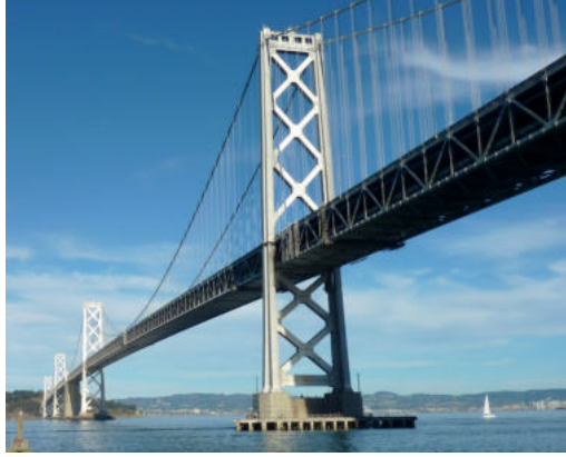
Figure 4: San Francisco–Oakland Bay Bridge in California, USA. Source [90].
