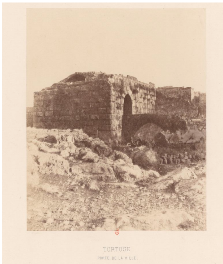
Figure 9. The citadel gate tower around 1859. Source: Louis de Clercq, Voyage en Orient , pl. 12.
