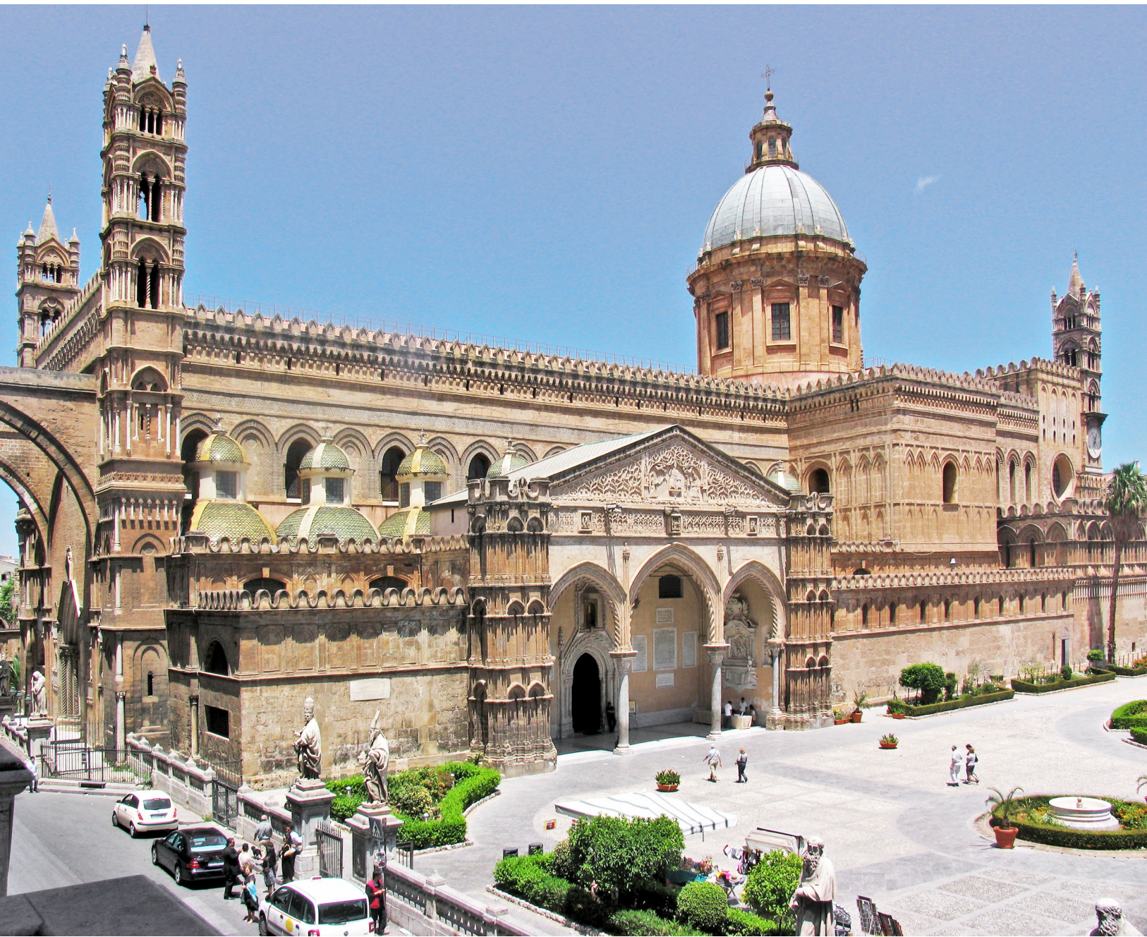
1/ Southern façade, with Antonino Gambara's portico (1453) and Ferdinando Fuga's dome (1801), Palermo Cathedral
